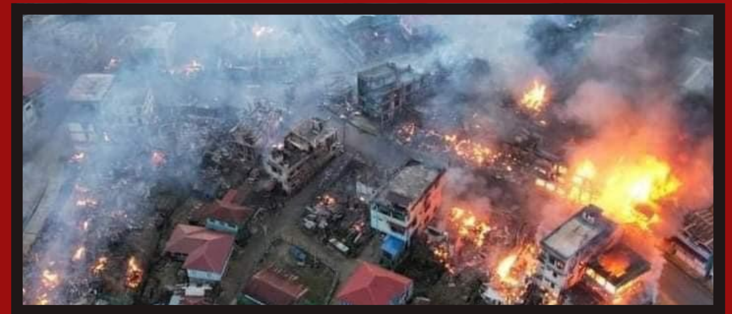
Thantlang Town, Chin State After Being Destroyed by the Junta
